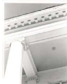
DENTIL WORK ON THE ROOF SOFFIT AND THE TOP OF A COLUMN.
